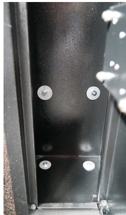
Show all anchor points. A minimum of two anchorage bolts into two separate immovable surfaces ie floor and wall is required
